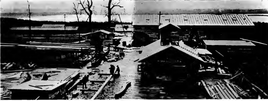
General view of the shops at the Standifer-Clarkson shipyard. An extensive building program is keeping this firm running at full capacity.
